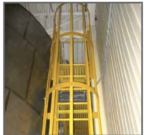
Ladder with Walk-thru and Rail Connections to Floor
