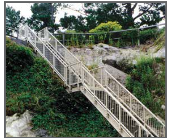
This all FRP stairway is located at a private residence in the Pebble Beach community in California. The stairway leads from the front yard of the home to the private beach below.
