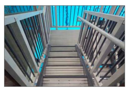
For the safety of aquatic centre users, Aqua Grate<sup>®</sup> Pultruded Grating, a non-slip and corrosion resistant grating, was installed to replace the rusted steel, allowing for optimum comfort under bare feet - a must in high traffic public recreational areas. Fibergrate's Dynarail<sup>®</sup> modular handrail system was also integrated on each side of the walkways and platforms for additional safety.
