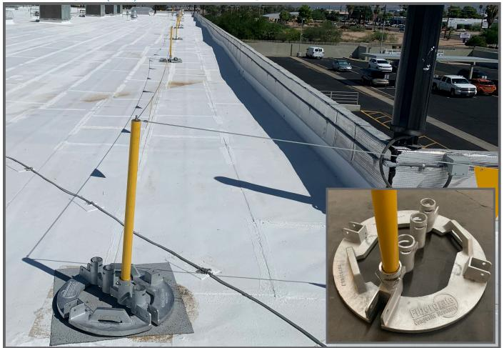
This permanent warning system includes heavy-duty base plates, plastic coated cable and rigid, plastic pennants. The heavy-duty stanchions and bases are designed to withstand years of use. The standard system includes 3 stanchions, 3 bases, and 100 feet of cable with plastic flags.
